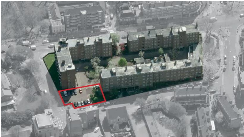
Aerial site location
